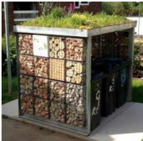
A bin store with green roof and habitat features
